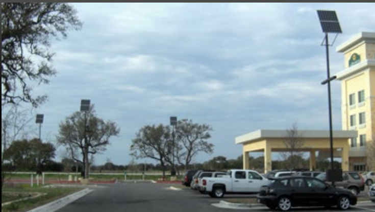
La Quinta Hotel Car Park - Solar Assist
