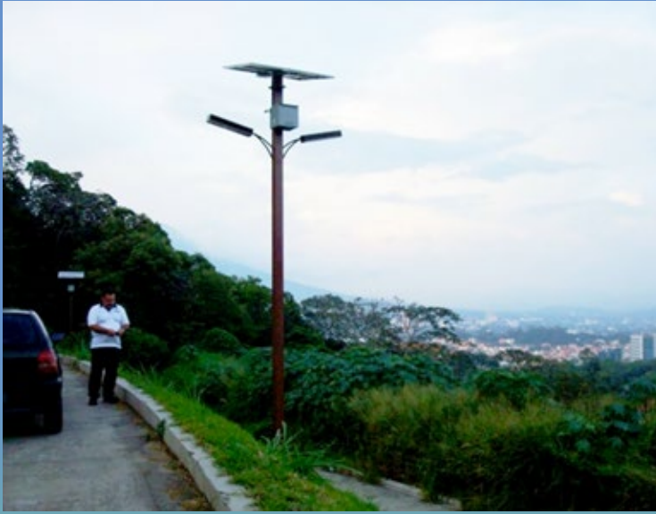
Solar Only Road and Walkway - El Salvador
