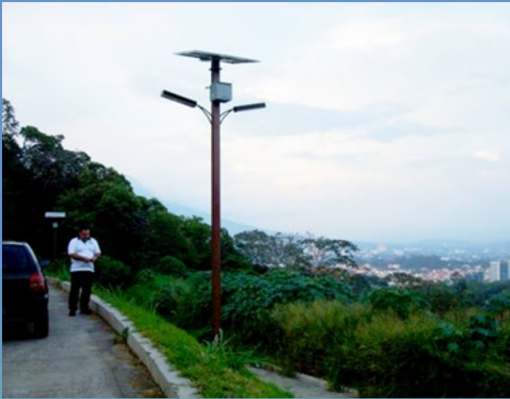
Solar Only Road and Walkway - El Salvador
