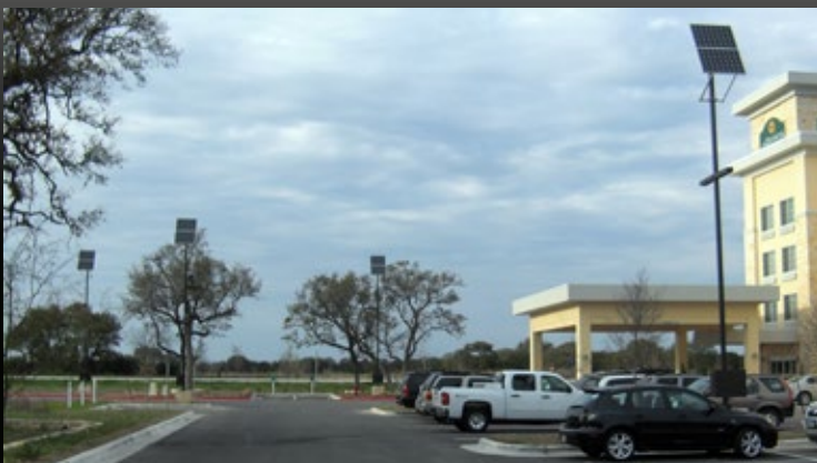
La Quinta Hotel Car Park - Solar Assist
